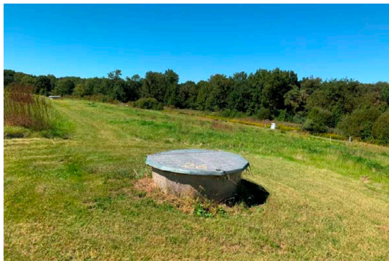
Photo #4 – Methane Well – top of landfill cap
