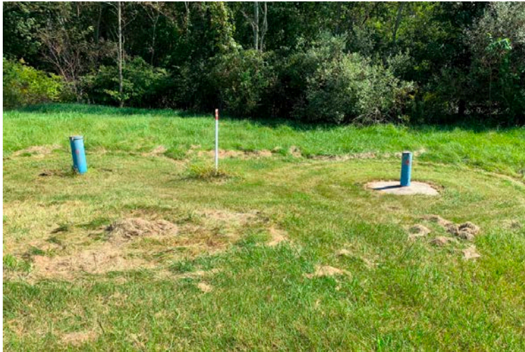
Photo #3 – Monitoring Wells – edge of landfill cap
