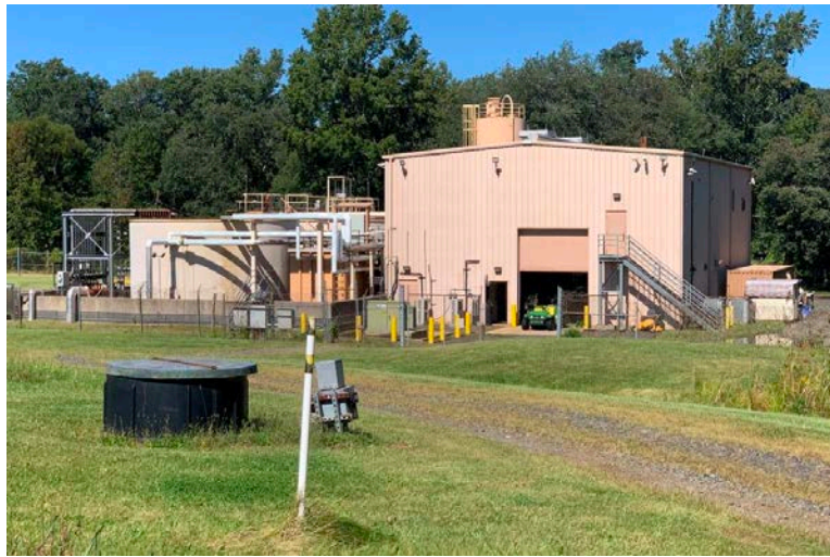
Photo #2 – Remediation / Maintenance building; wastewater treatment plant
